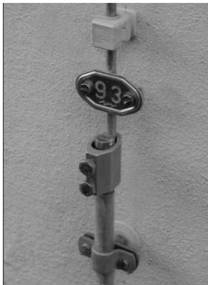
Test joint with disconnecting sleeve
